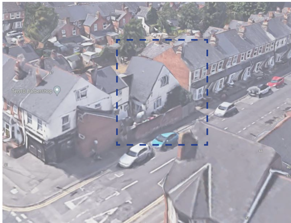
Beresford Road end of terrace development
