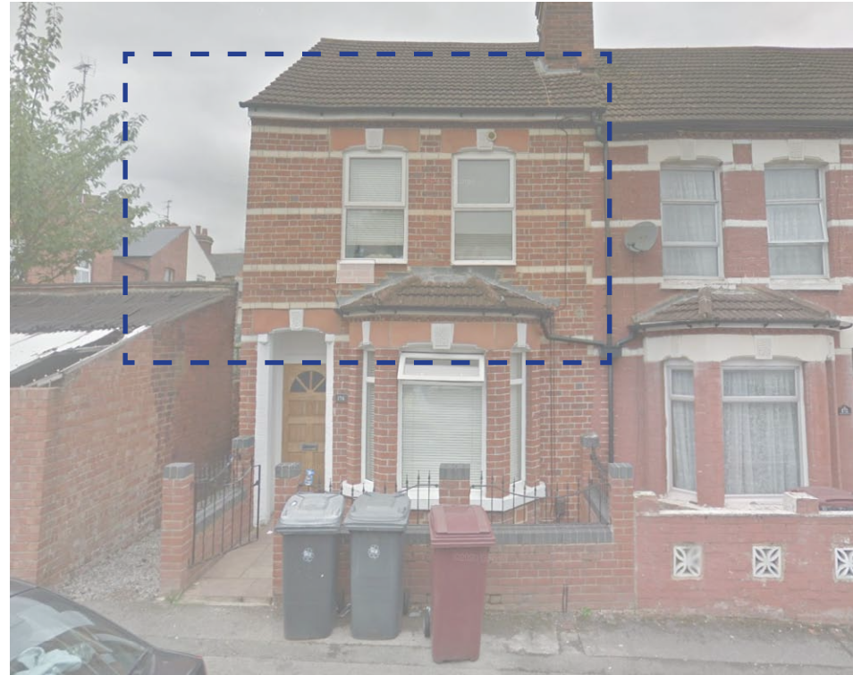
Adjoining property exhibits a mix of red brick and buff brick pattern banding
