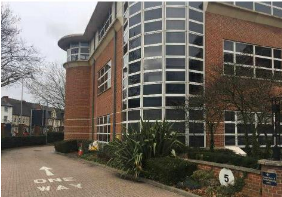
South facing car park from walkaround photos showing scale of existing building in relation to neighbouring houses
