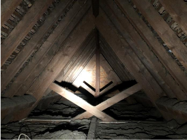
Photograph 7. Loft void 1 of Building 1.
