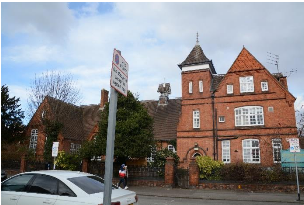
Photograph 3. The western side of the southern elevation of Building 1.
