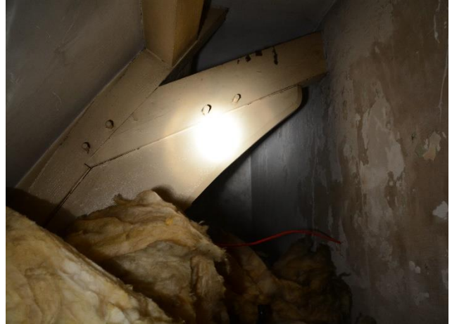
Photograph 8. Loft void 2 of Building 1.
