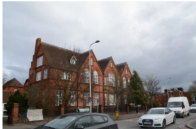
Photograph 4. The eastern side of the southern elevation of Building 1.
