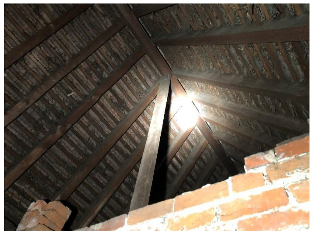
Photograph 6. Loft void 1 of Building 1.
