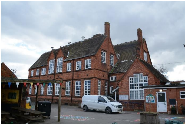
Photograph 1. The eastern side of the northern elevation of Building 1.
