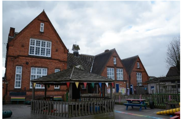
Photograph 2. The western side of the northern elevation of Building 1.
