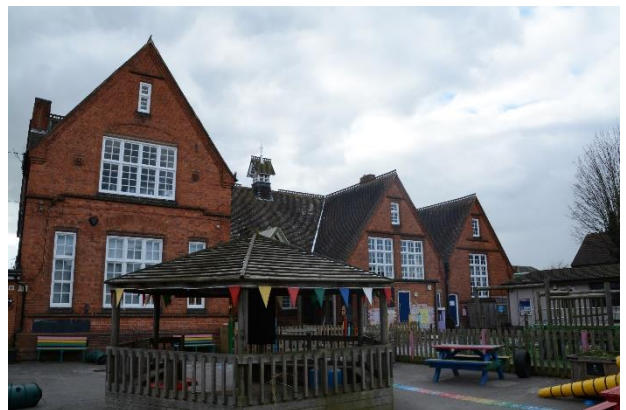
Photograph 10. The northern elevation of Building 5.
