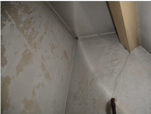
Photograph 7. Loft void 2 of Building 1.
