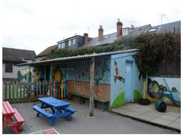
Photograph 8. The southern elevation of Building 3.
