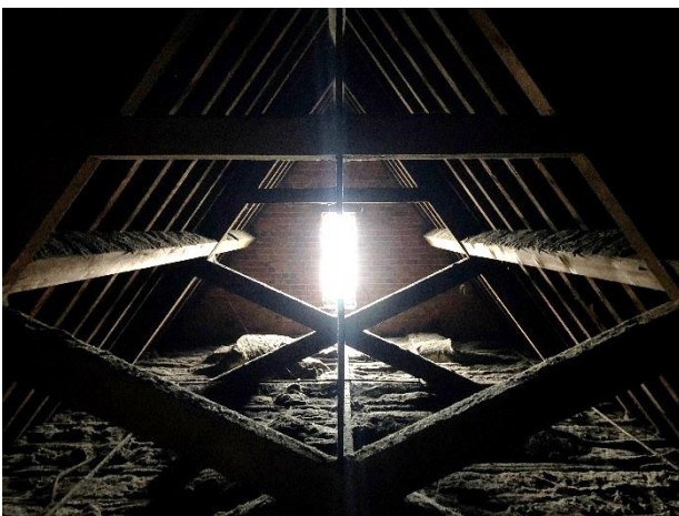
Photograph 5. Loft void 1 of Building 1.
