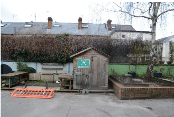
Photograph 9. The southern elevation of Building 4.
