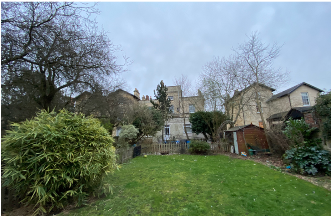
Fig.8: Existing rear view of 9 Eldon Square & garden
