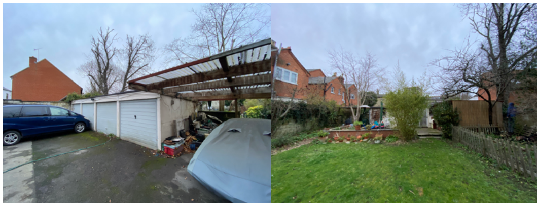
Fig.3: (left) Existing views of existing garages and car-port structure & Fig.4: (right) Existing view of 9 Eldon Square garden, facing towards existing garages
