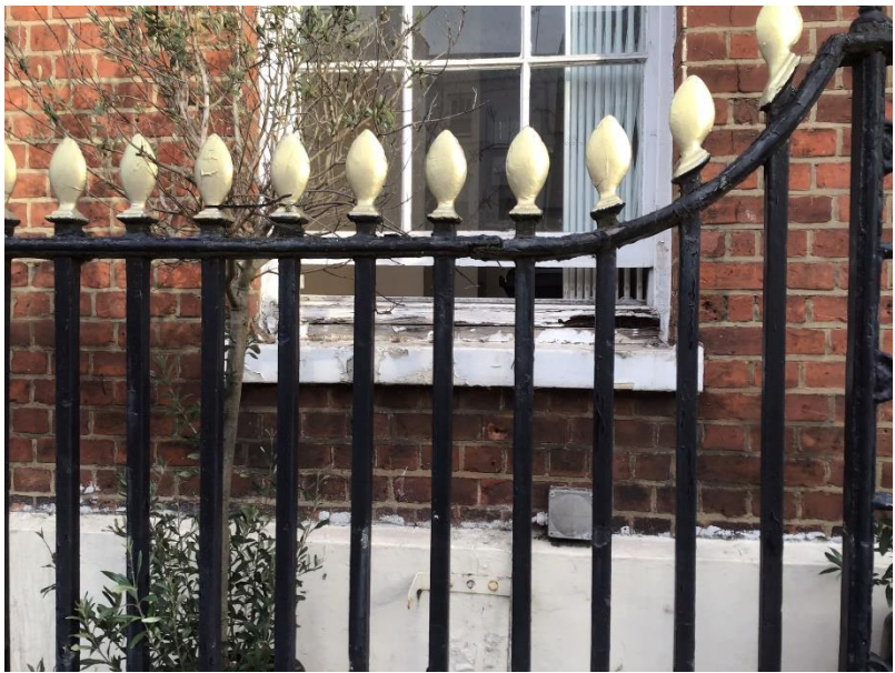
Rotten box sash on ground floor.
