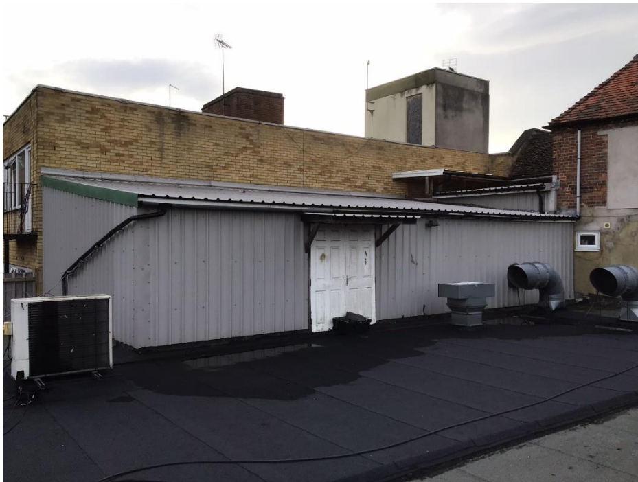
Various area s of roof repairs.
