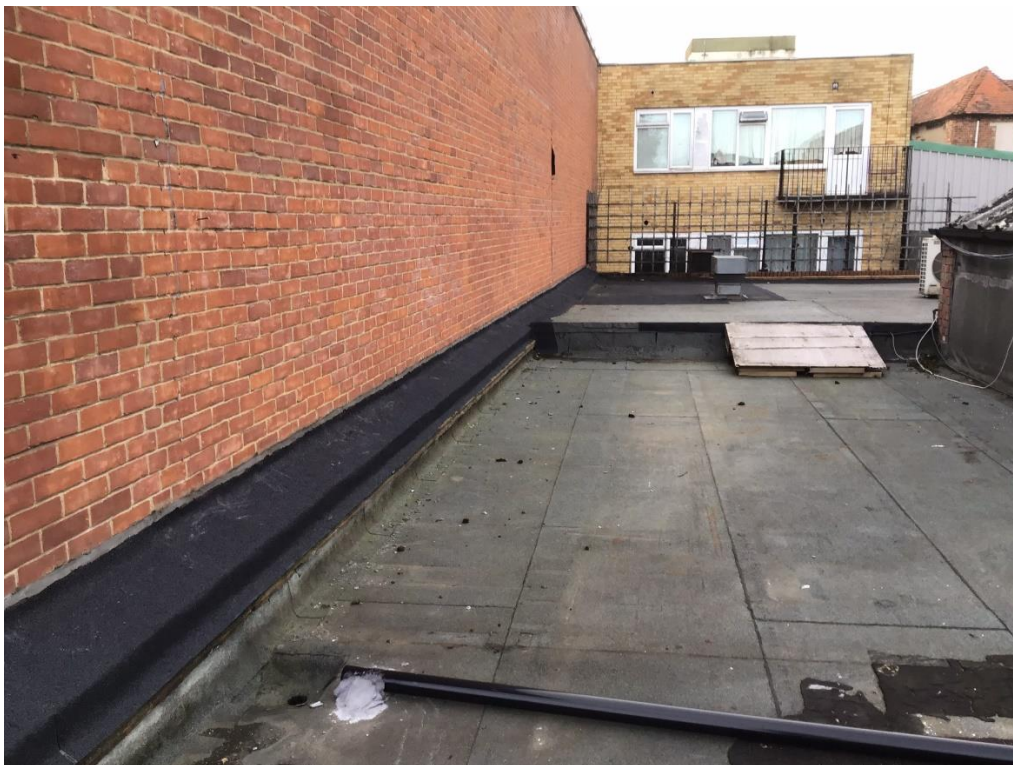
View of the left hand flat roof section looking from the rear showing repaired sections.
