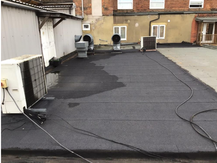
Various areas of roof repairs
