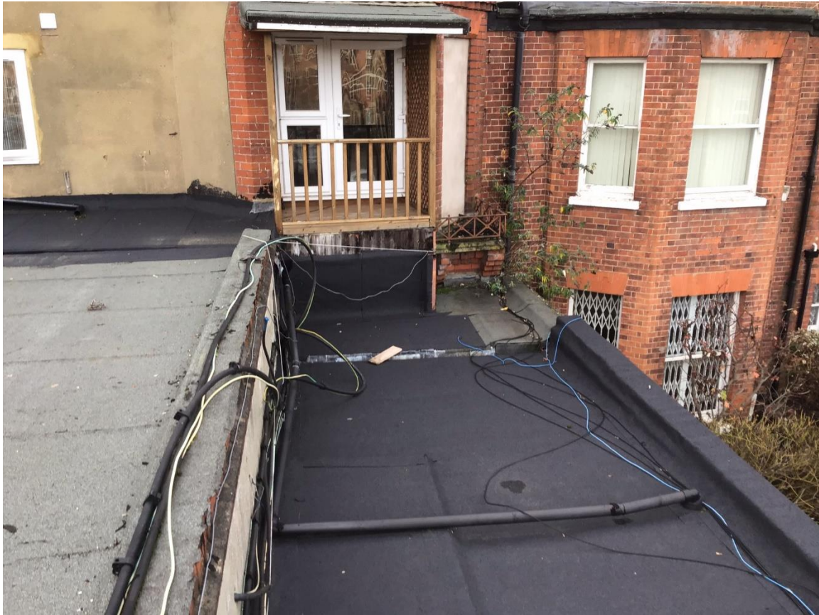
Various areas of roof repairs.
