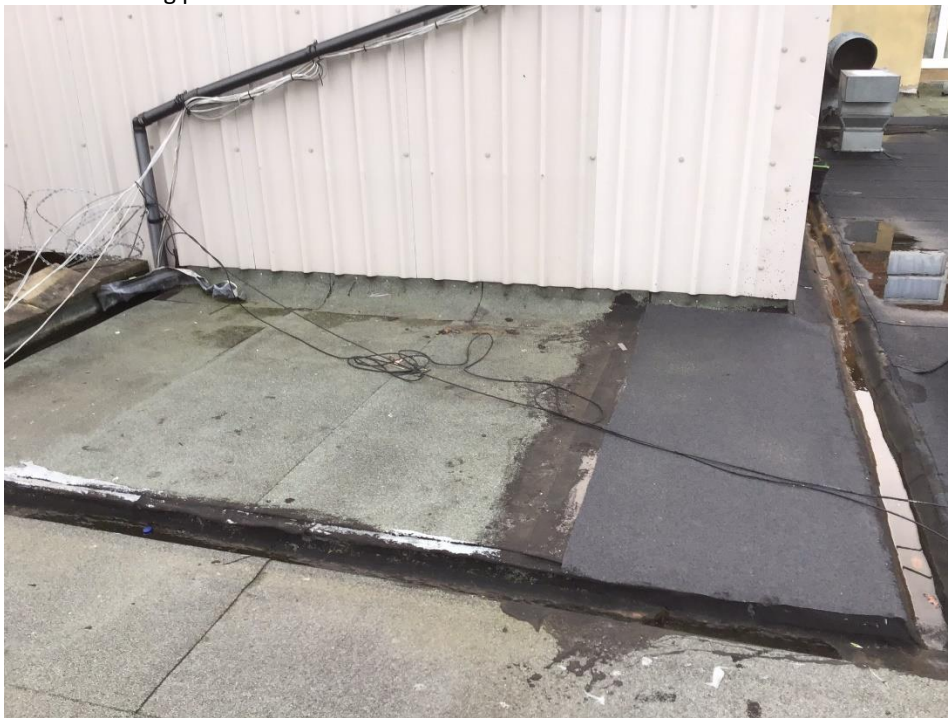
Various sections of roof repairs.
