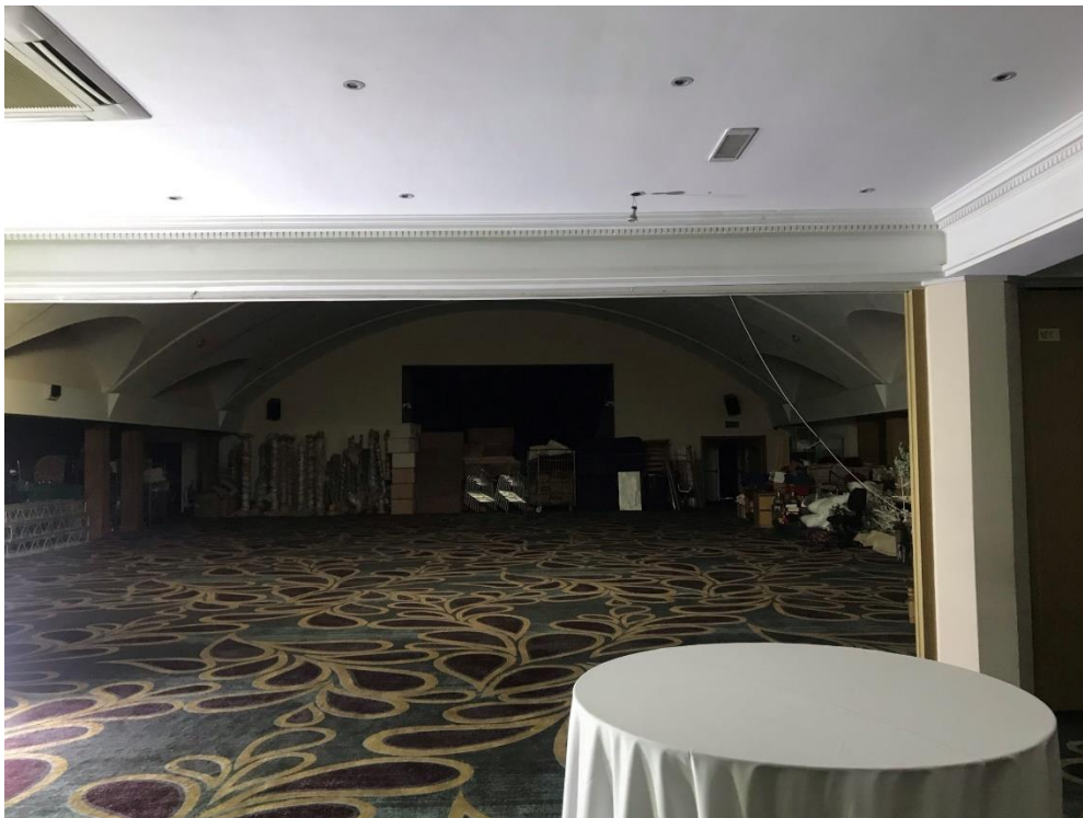
View of main dance floor under corrugated pitch roof
