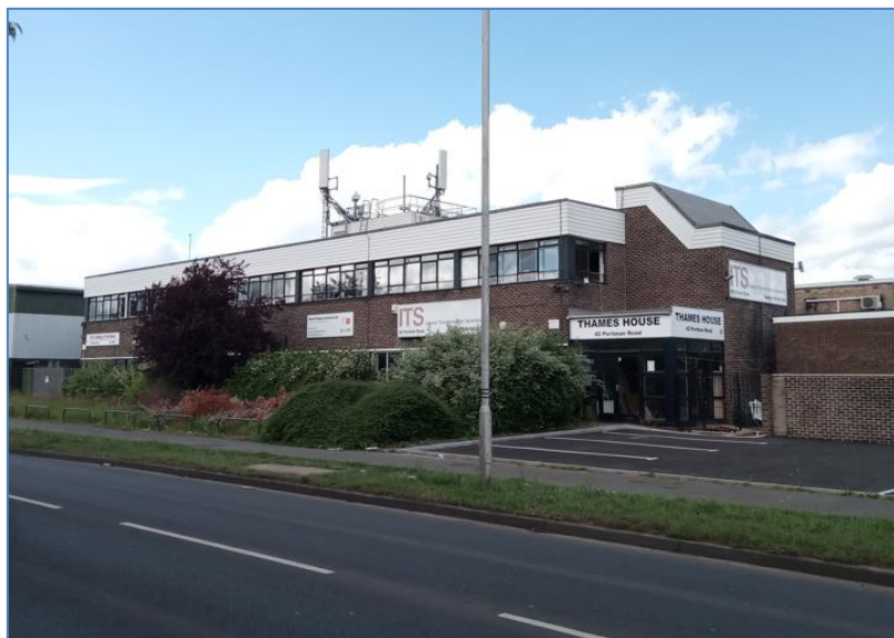
Fig 1. Front of 42 Portman Road. Photo taken by case officer on 20/05/2022
