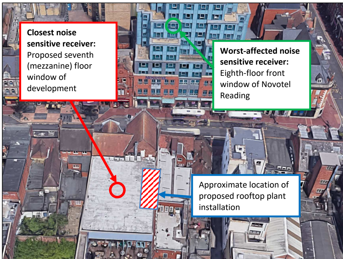
Figure 6.2 Closest noise sensitive receivers relative to plant installation (Image Source: Google Maps)
