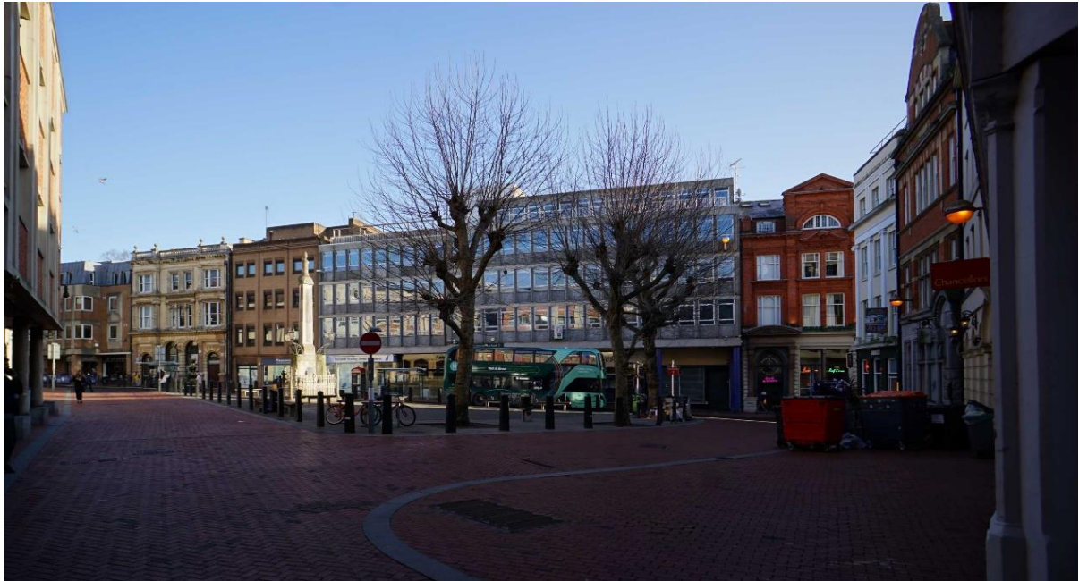
Figure 17: View of the application site from the south-west across Market Place. The large 1960s facade is at odds with the historic character of the public square in scale, material and articulation.
