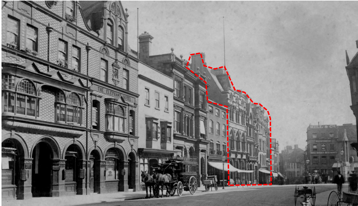
Figure 23: Photograph 1890 looking south along the west side of Market Place. Like the application site in the background, the Victorian, Elephant Hotel on the left was developed in the 1960s
