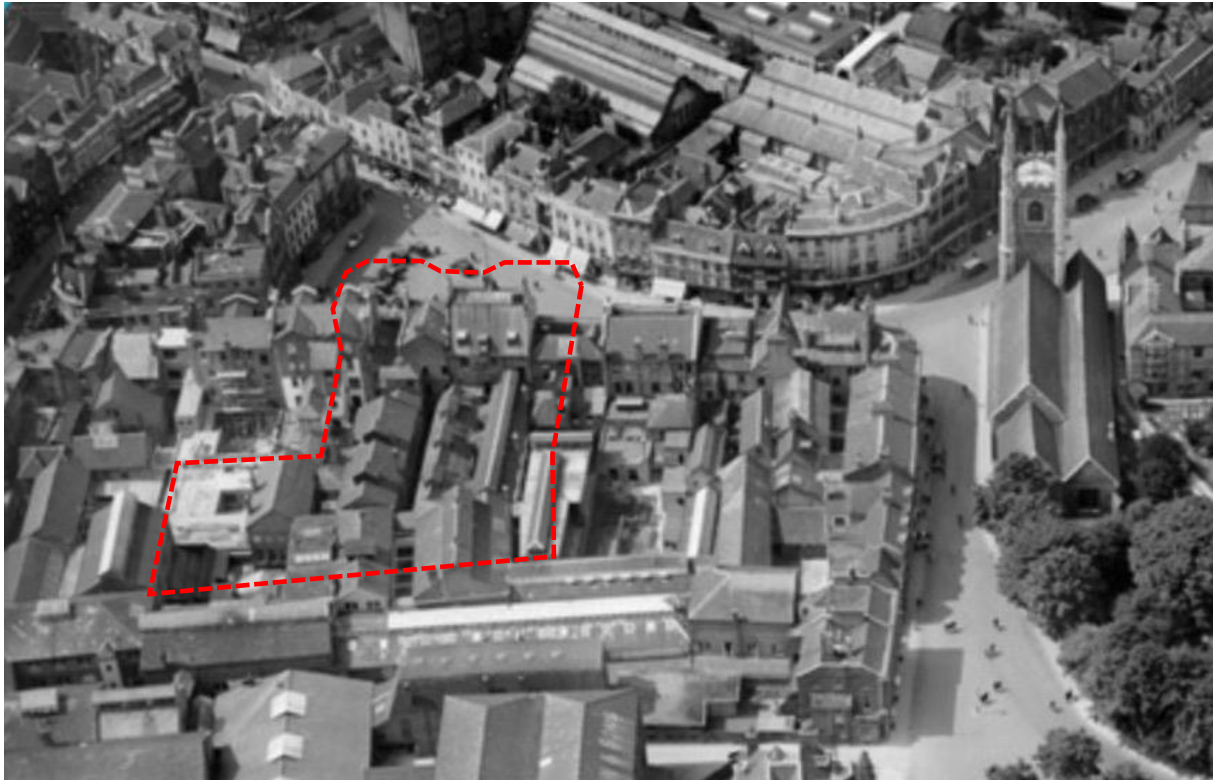
Figure 26: Aerial photograph from 1928 providing a good view of the difference between the polite market facing buildings and the industrial rear. This pattern is apparent on both east and west sides of Market Place.
