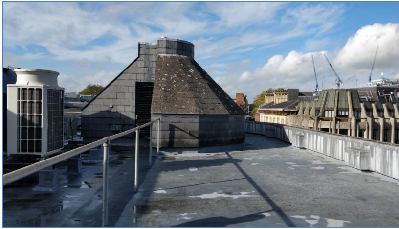
Photo 2: Exterior of the plant room on flat roof of main building
