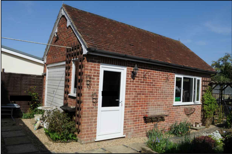
PHOTO OF GARAGE TO BE DEMOLISHED
