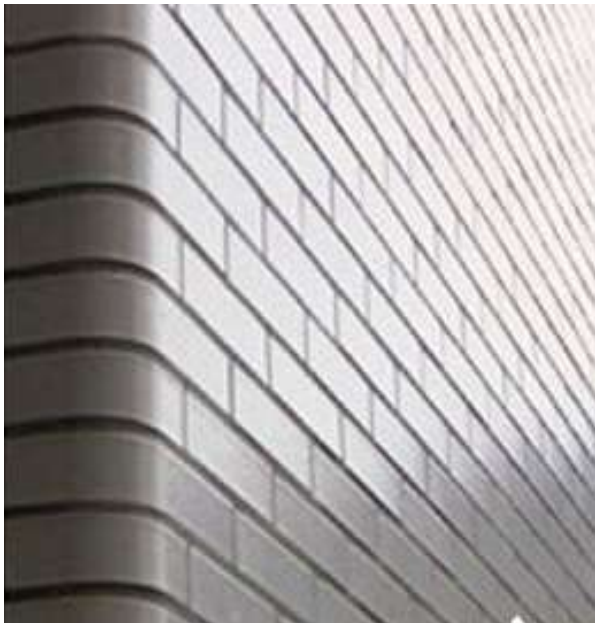
White glazed brick to balcony recesses
