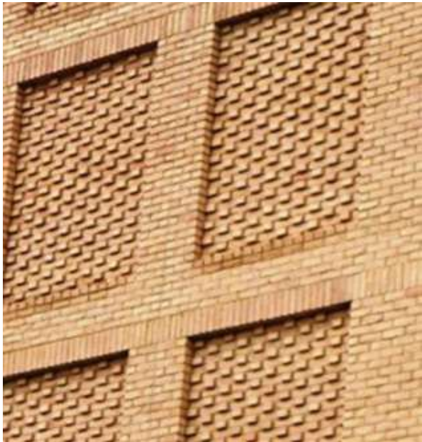
Recessed brick panels with patternated brickwork
