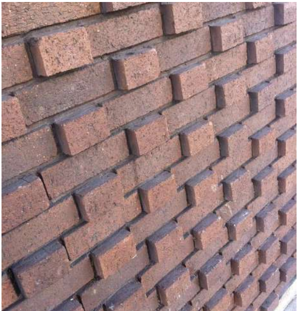
Patternated brick work
