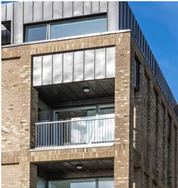
Recessed corner balconies
