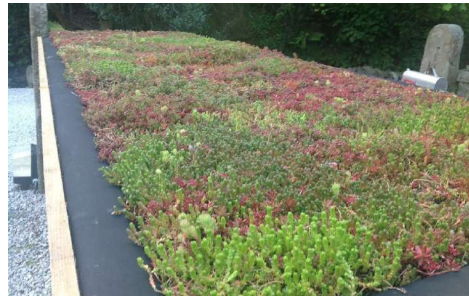
Green Sedum roof
