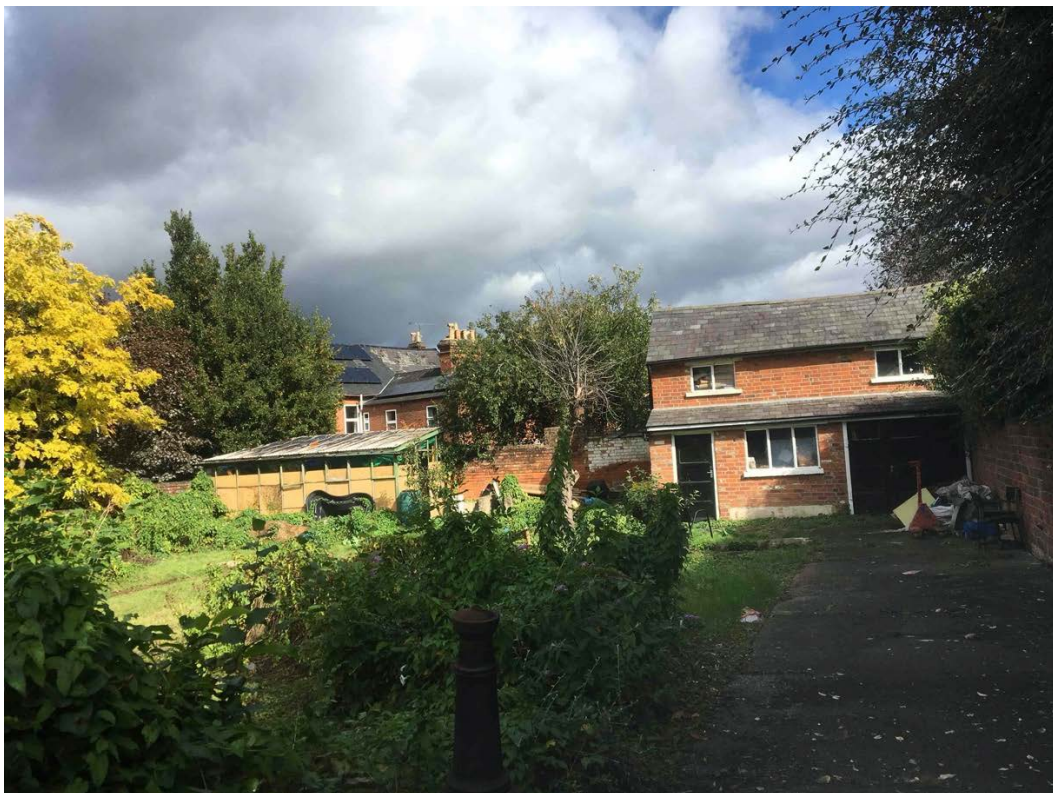
Coach House Storage Shed
