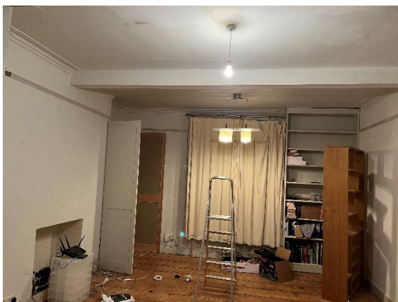
Photograph: 6 Level: Ground Floor View: Front facing reception room Element: Drop ceiling bulkhead
