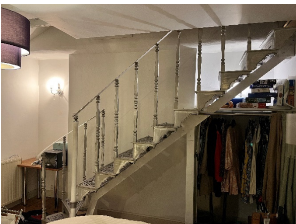
Photograph: 9 Level: First Floor View: From bedroom 1 Element: Staircase accessing the roof space
