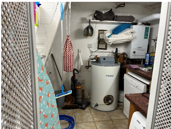
Photograph: 4 Level: Basement View: From kitchen into Utility Room Element: Space to be reconfigured and improved
