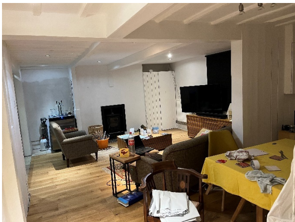
Photograph: 1 Level: Basement View: From Bottom of Staircase into dining/living area Element: Opening to be infilled to create 2.no separate areas
