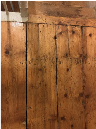
Photograph: 7 Level: First Floor View: Landing area Element: Exposed finish floorboards
