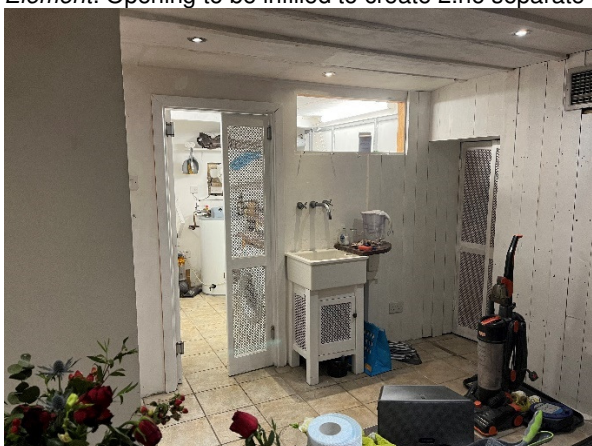
Photograph: 3 Level: Basement View: From kitchen into Utility Room Element: Opening to be infilled to create 2.no separate areas
