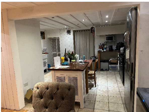
Photograph: 2 Level: Basement View: From living room into kitchen Element: Opening to be infilled to create 2.no separate areas
