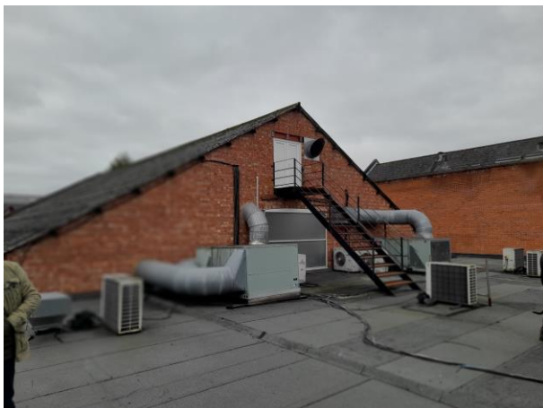
Photos 4, 5 and 6 Rooftop views.
