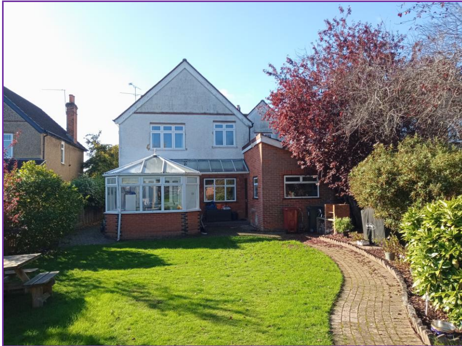
Figure 2: Existing Rear Elevation
