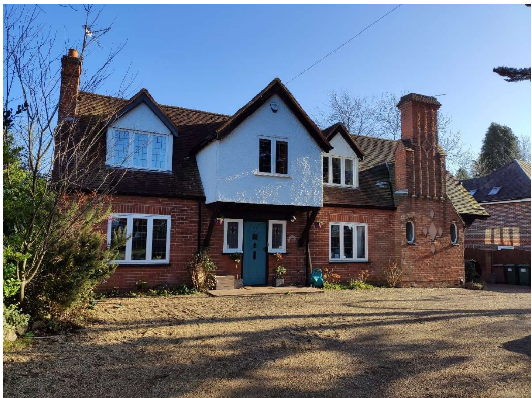
Site – Existing house viewed from the road
