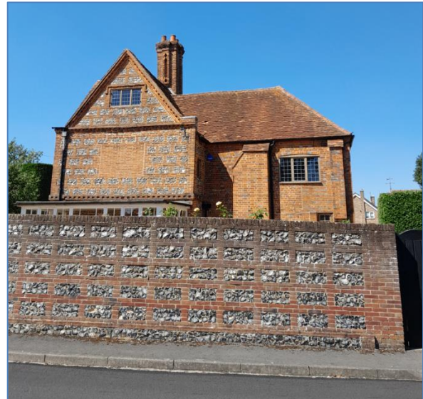
Fig 2. Side of Old Grove House. Photo taken by case officer on 11/08/2022
