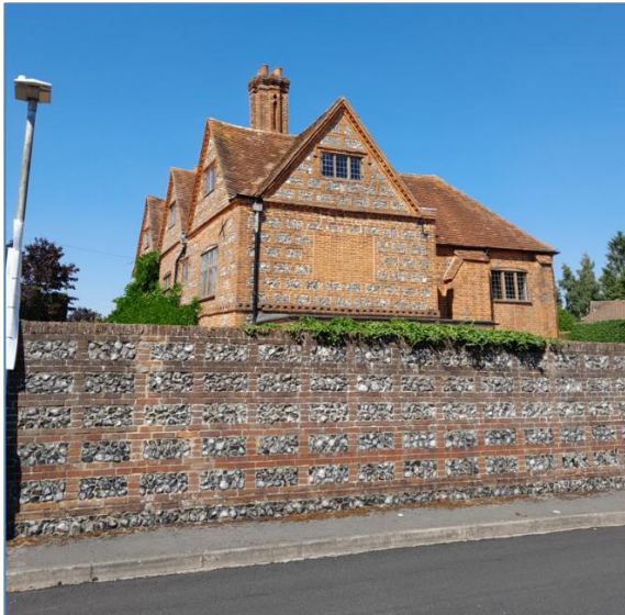
Fig 1. Side of Old Grove House. Photo taken by case officer on 11/08/2022
