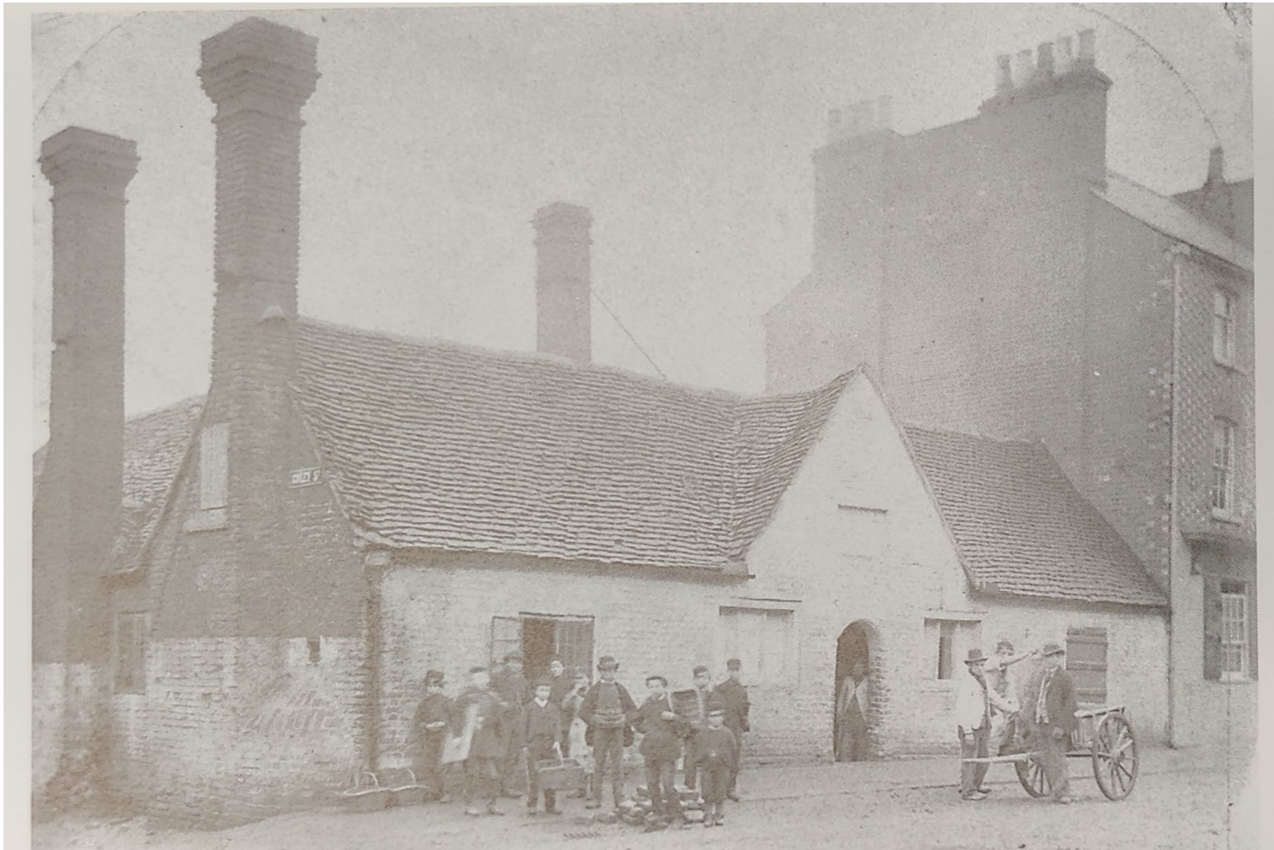
Figure 15 c. 1870 – Vachel Almshouses at the junction of Coley Street and Castle Street
