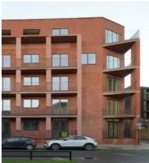
Precedent Building loggia and general needs amenity space
