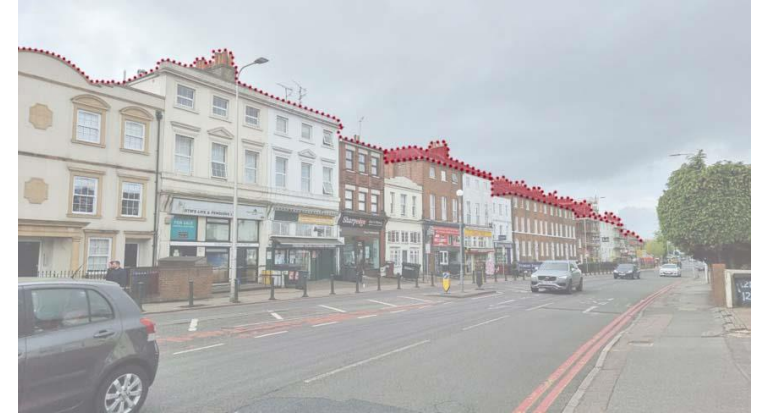
Pitched, parapet and flat roofs along Oxford Street-Limited visibility of pitched roofs
