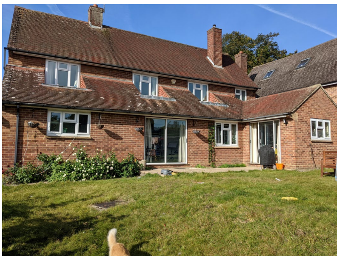
Current rear view of the property
