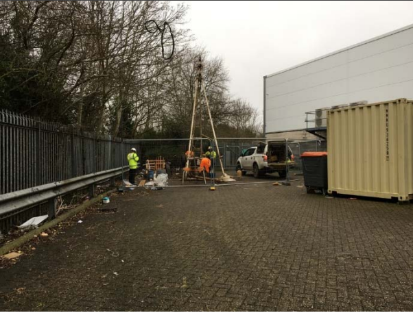
17: Cable percussive rig set up
