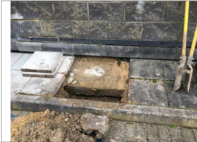
13: Exposed concrete beam
