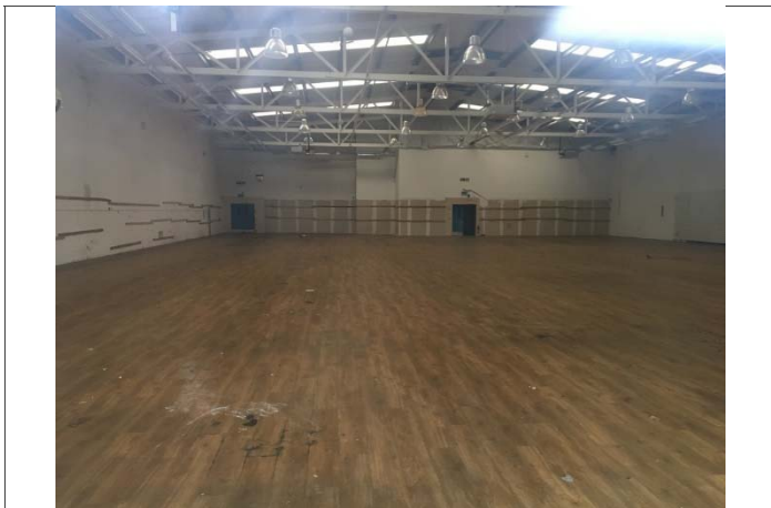
11: Internal Photograph of Unit 4
