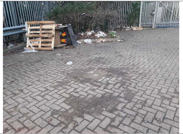
20: Example of reinstated position
