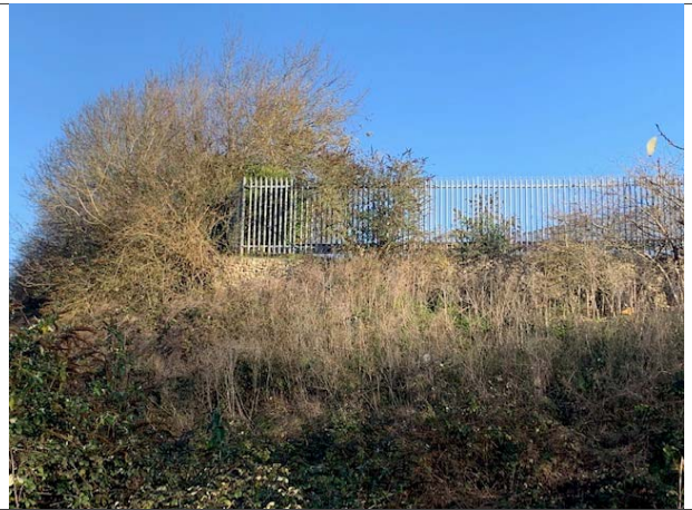
24: Overview of slope
