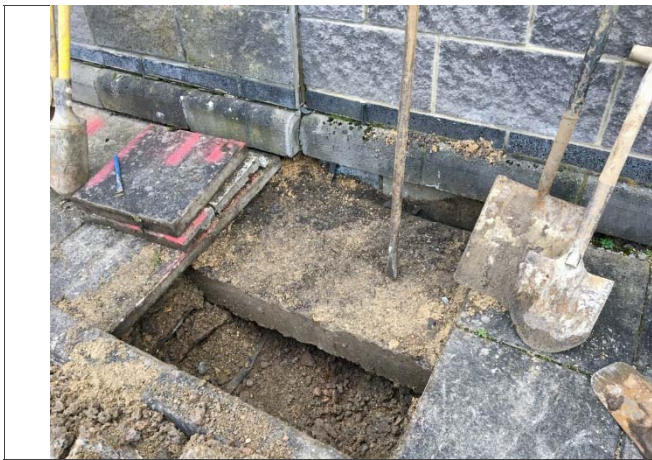
15: Continuation of concrete beam
