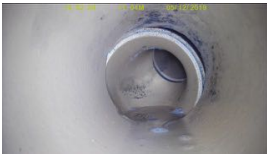
Displaced joint
