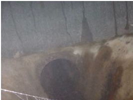
Displaced joint Section SW 17
