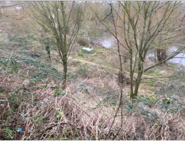
21: Overview of slope
