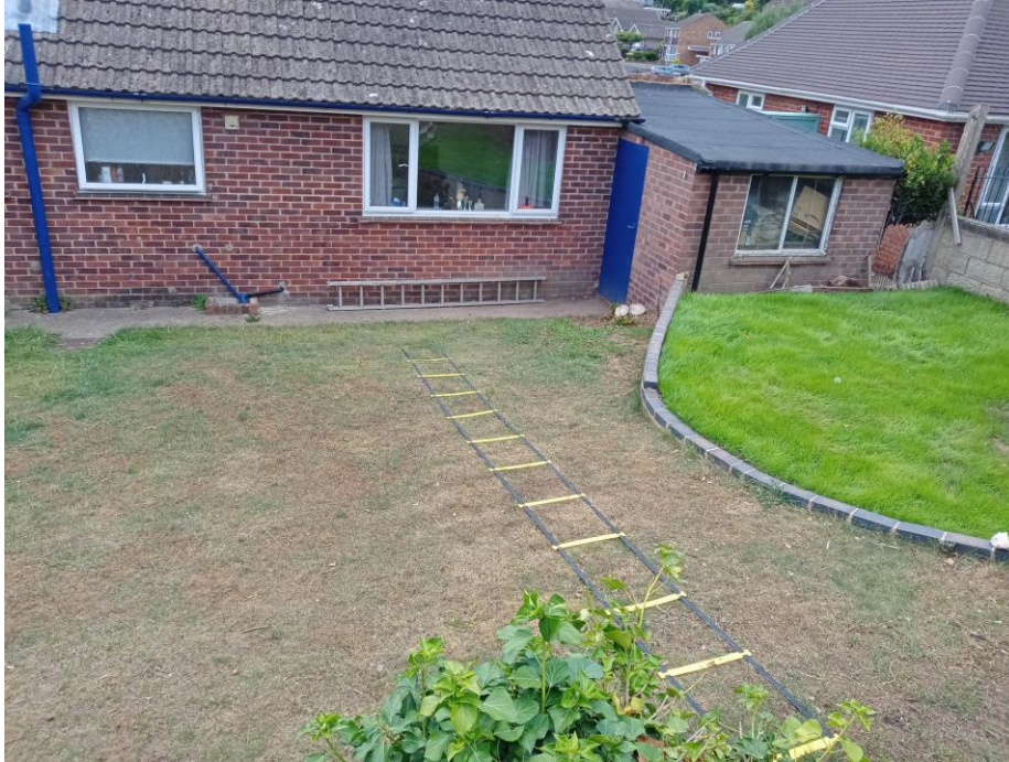
Figure 2: Existing Rear Elevation
