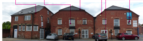
FORMER BREWERY BUILDING - INTERNAL FACADE
