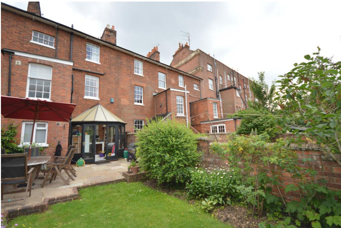
Pic 2. Existing conservatory to be removed.
