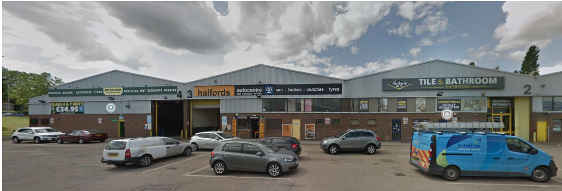
Figure 3: Stadium Trade and Business Park as existing, Unit 2,3 &4 in the foreground (South-East Elevation).
