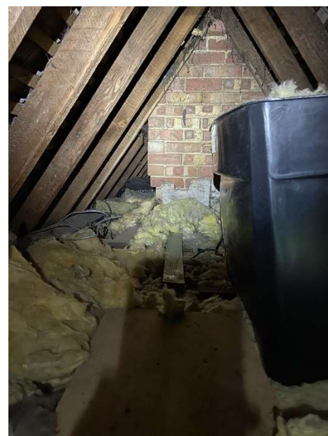
Photo 8: The southern part of the loft void in the building
