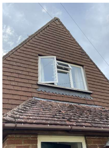
Photo 2: Front elevation of 5 Woods Road showing hanging tiles
