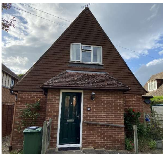
Photo 1: 5 Woods Road viewed from south east
