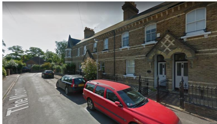
The stringcourse on the buildings diagonally across the road from 19 The Mount
