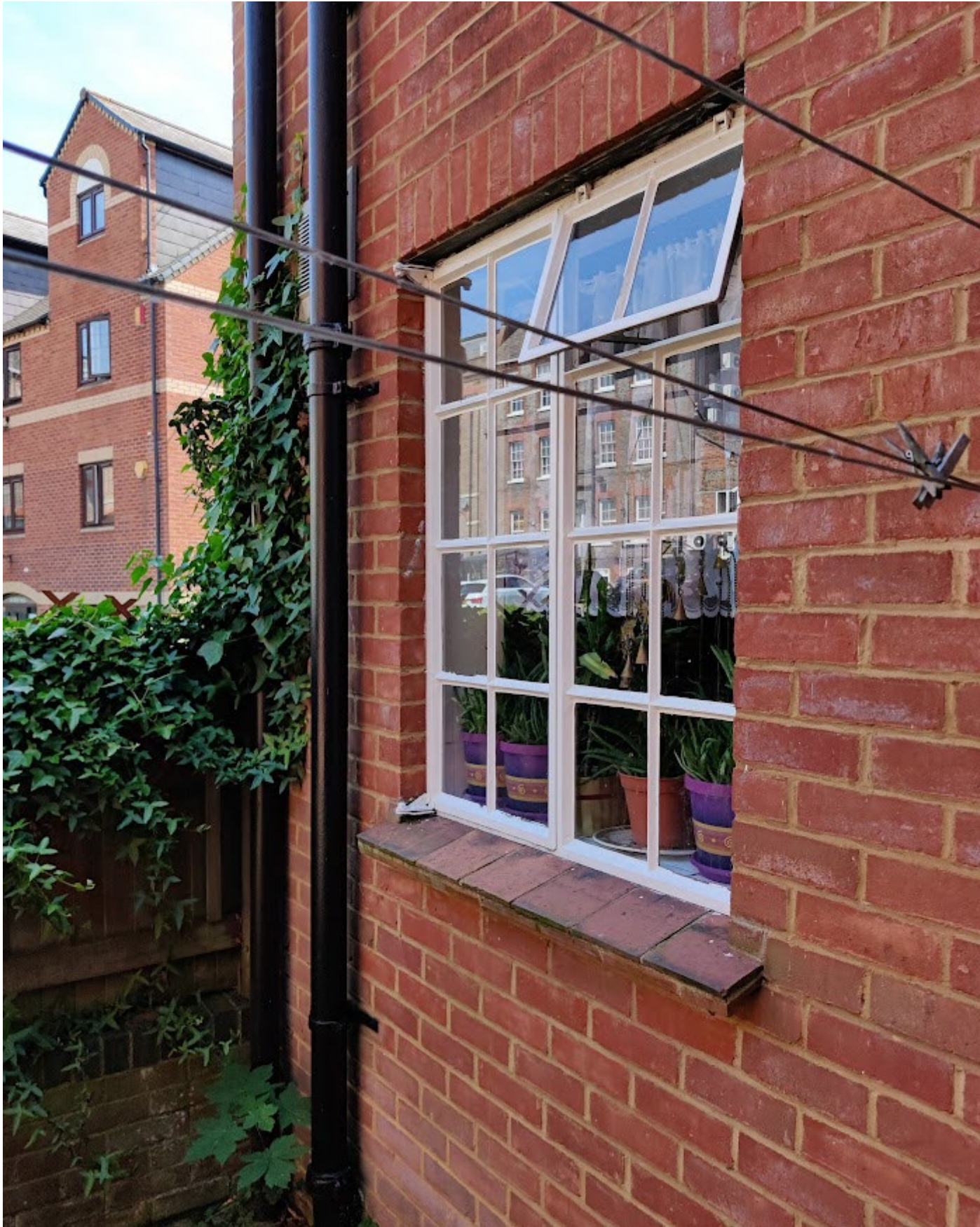
Figure 14. Typical Crittall windows to kitchens of East Wing
