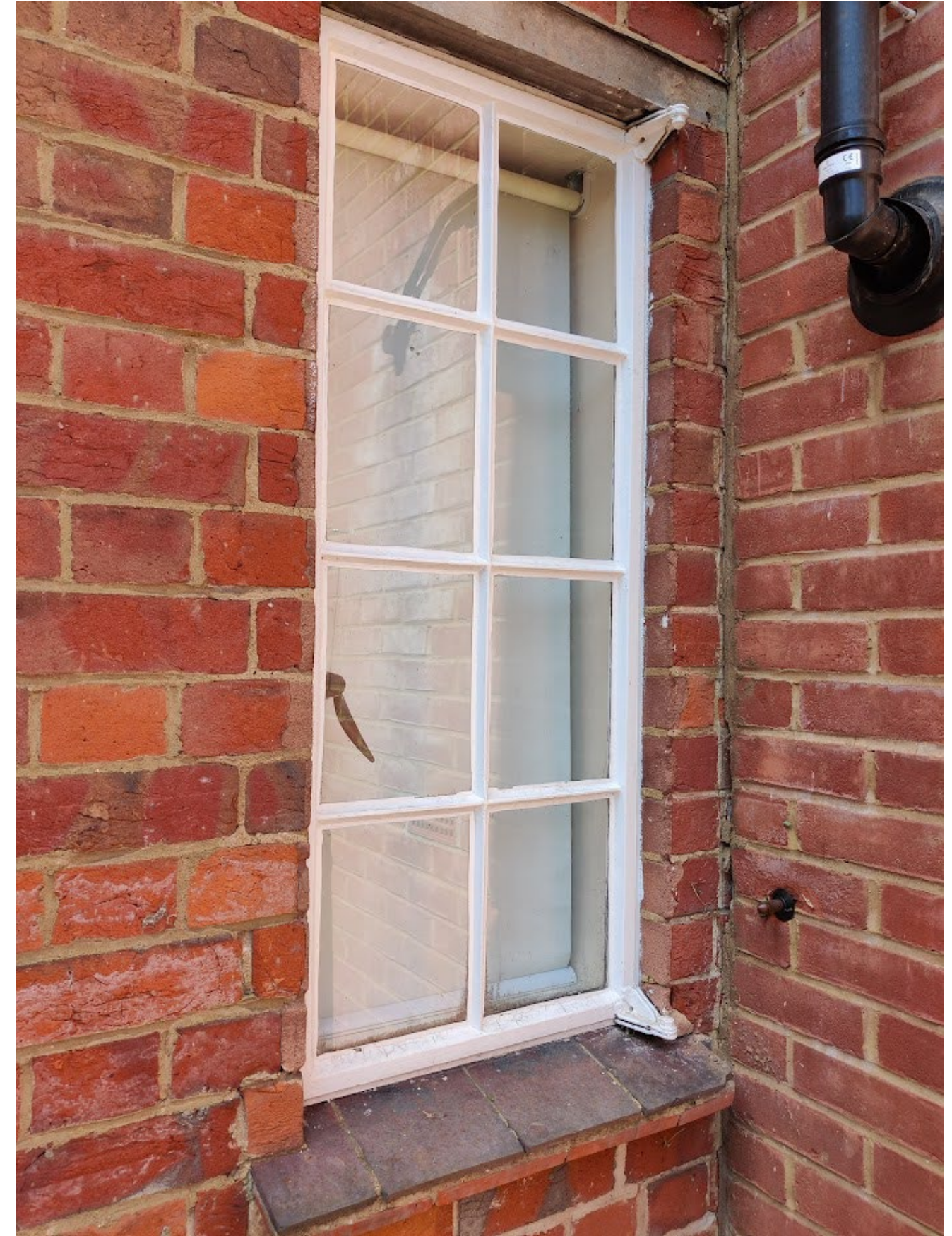
Figure 15. Typical Crittall windows to bathrooms and living spaces of the East Wing.
