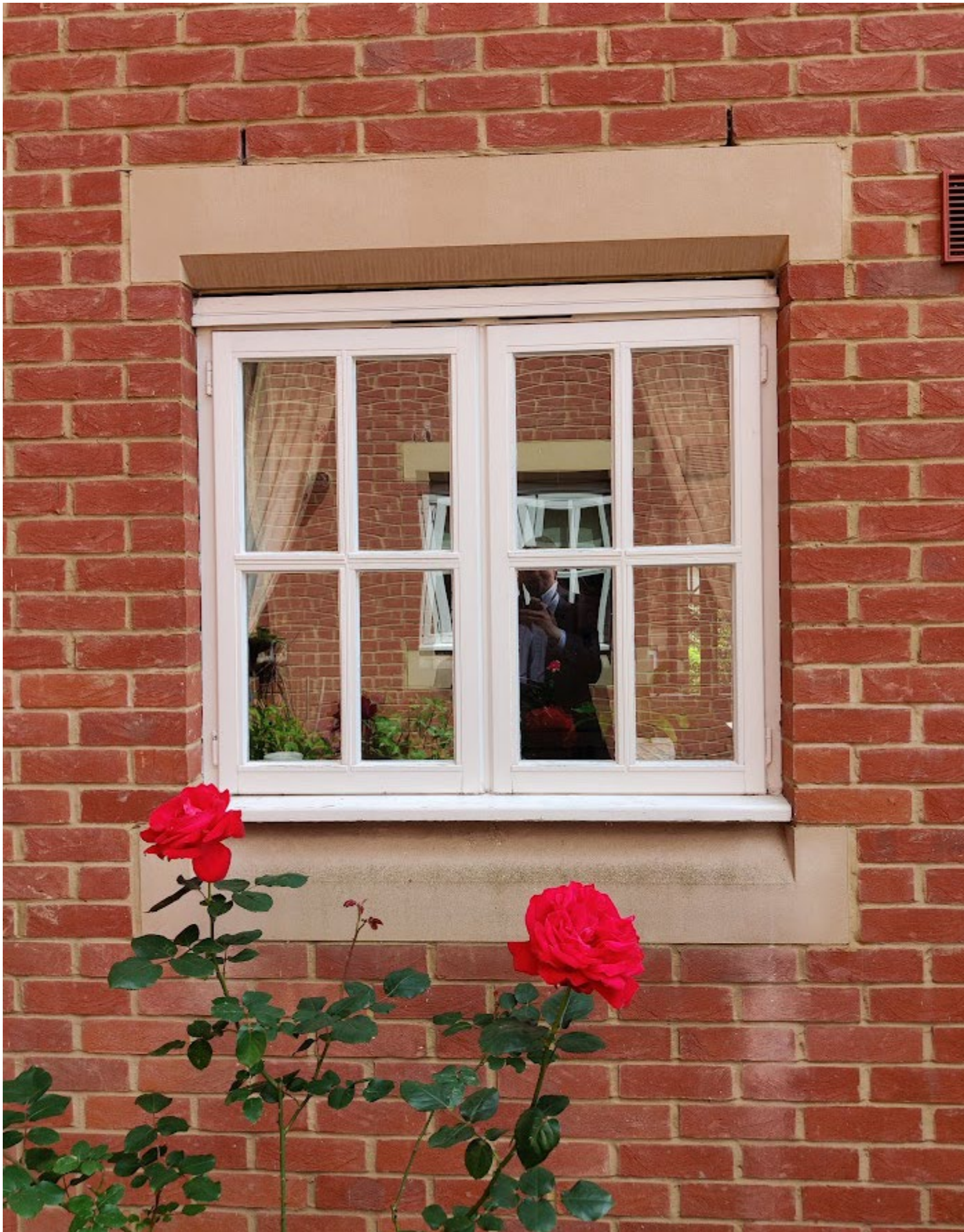
Figure 16. Typical double glazed timber windows to kitchens of Westt Wing
