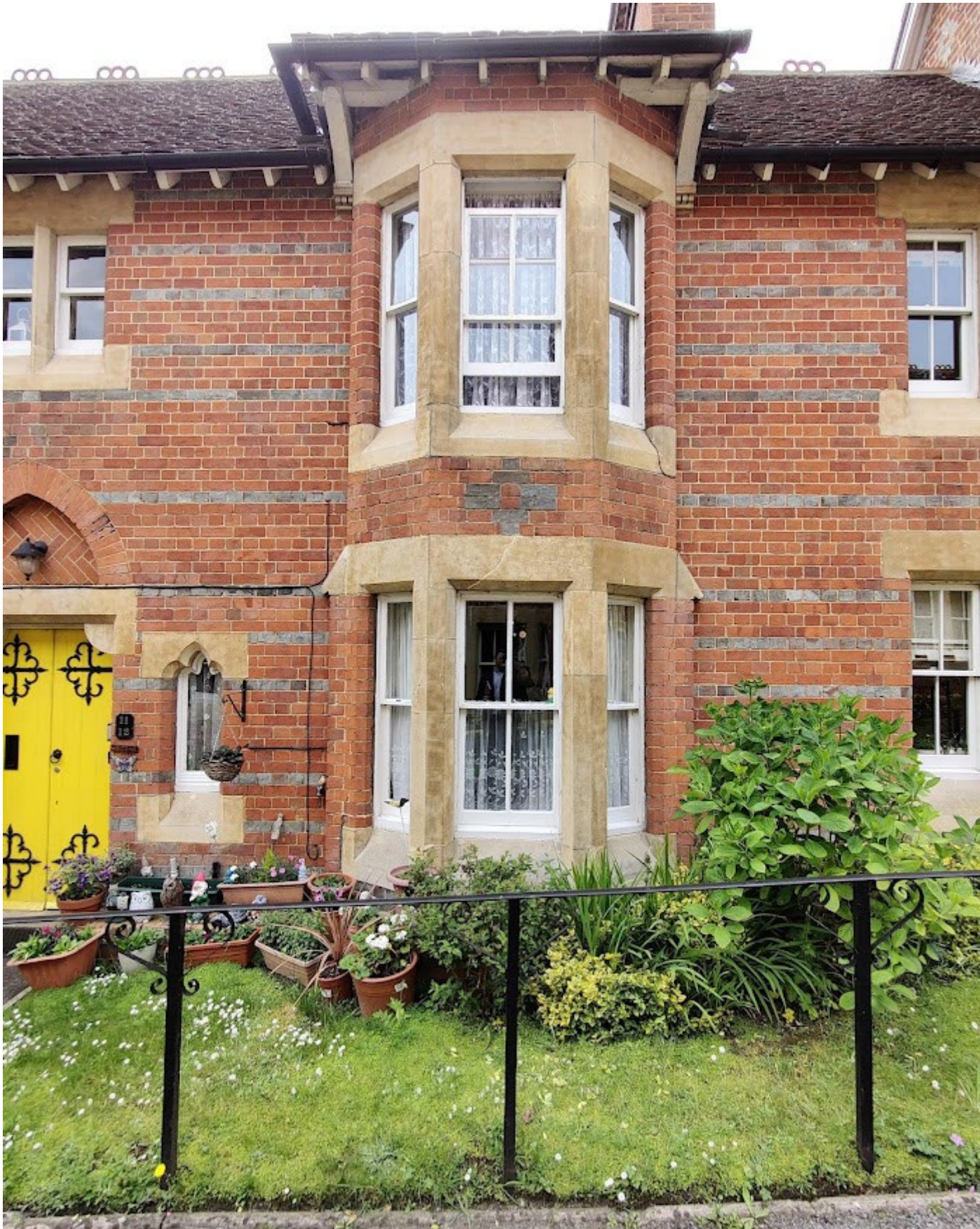
Figure 4. Typical 2 storey Bay Window
