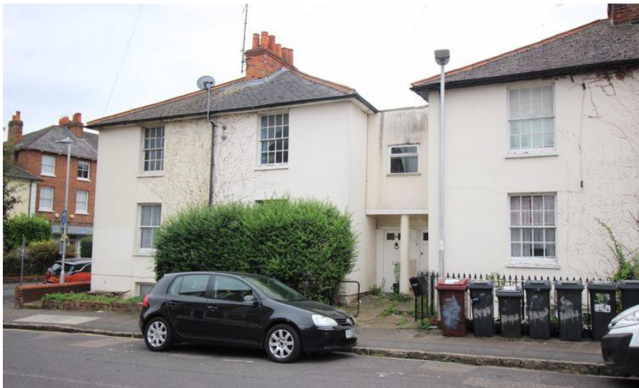
Plate 1: Front Elevation of No 33-37 Baker Street (No 35 has the hedge, window above door serves Bedroom 3)
