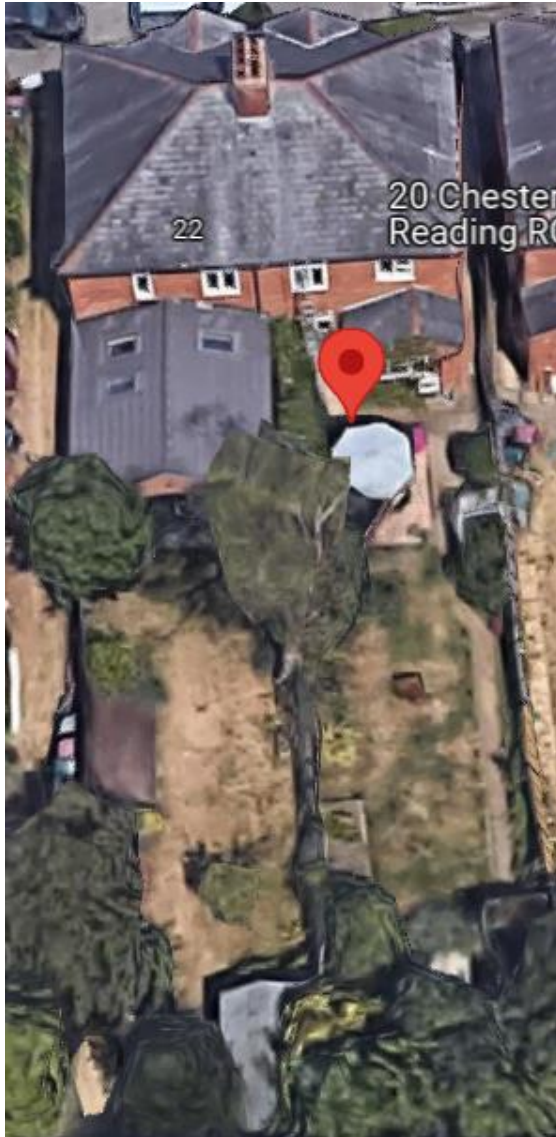
Fig 1: Aerial view of the site and the adjoining Semidetached dwelling (google image accessed 30/9/22)
