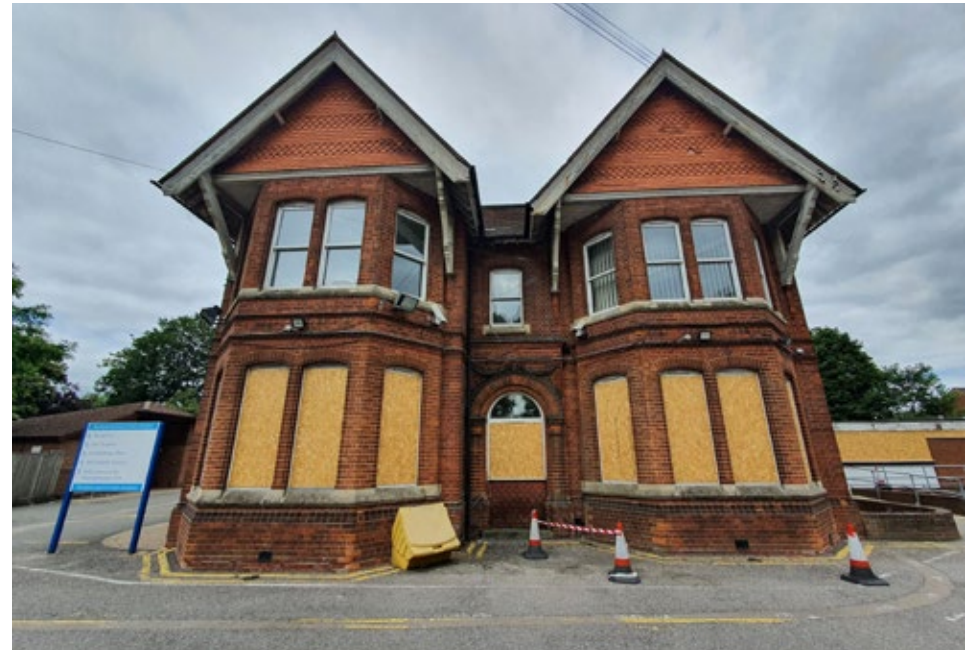
View of the front facade of the existing building
