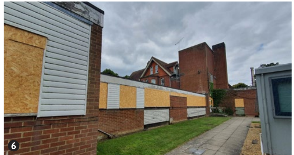
Rear of flat roofed extension
