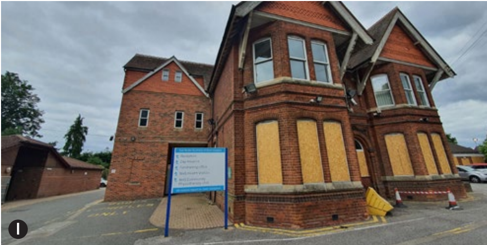
View of extension to historic building
