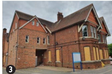
View of service entrance
