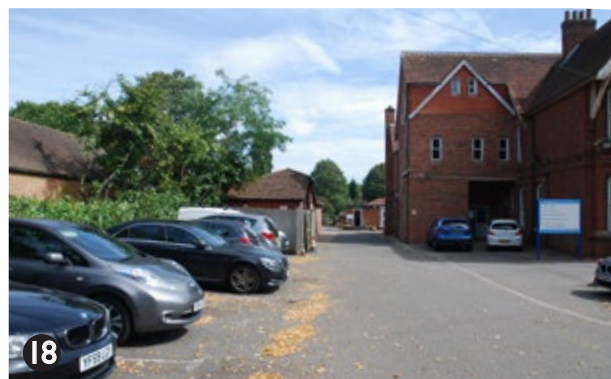
View east along access road adjacent to Block One
