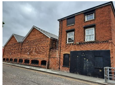
Plate 9.6: Office building in the west of the site – western elevation
