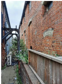
Plate 9.3: Disused warehouse in the east of the site – southern elevation
