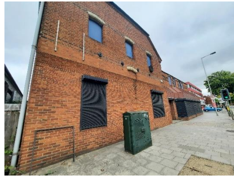
Plate 9.2: Disused warehouse in the east of the site – eastern elevation
