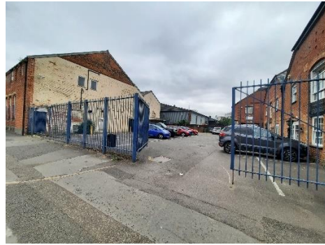
Plate 9.8: Metal palisade fence on northern site boundary
