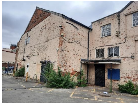
Plate 9.4: Disused warehouse in the east of the site – western elevation
