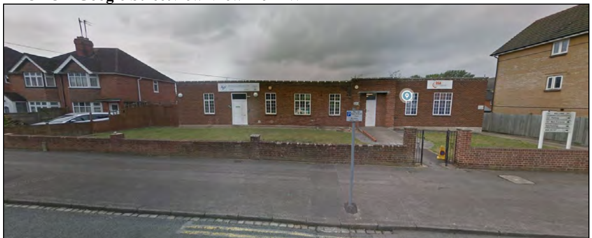
PHOTO 2 Google Streetview View from W
