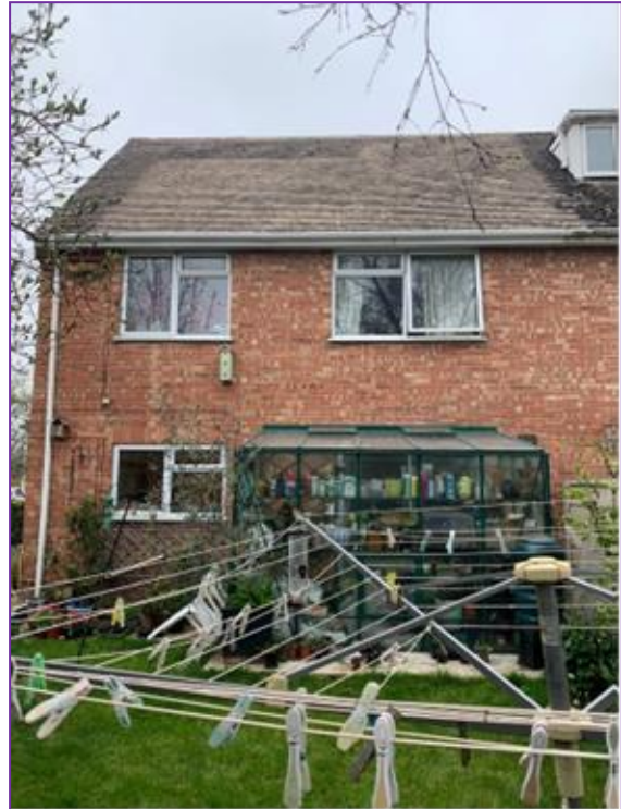
Fig 2. Existing Rear Elevation
