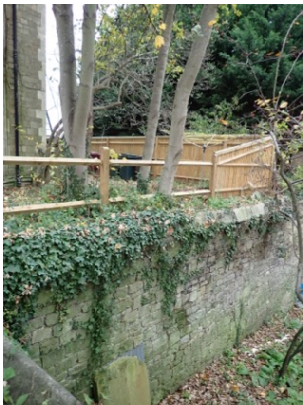
View of retaining wall.
