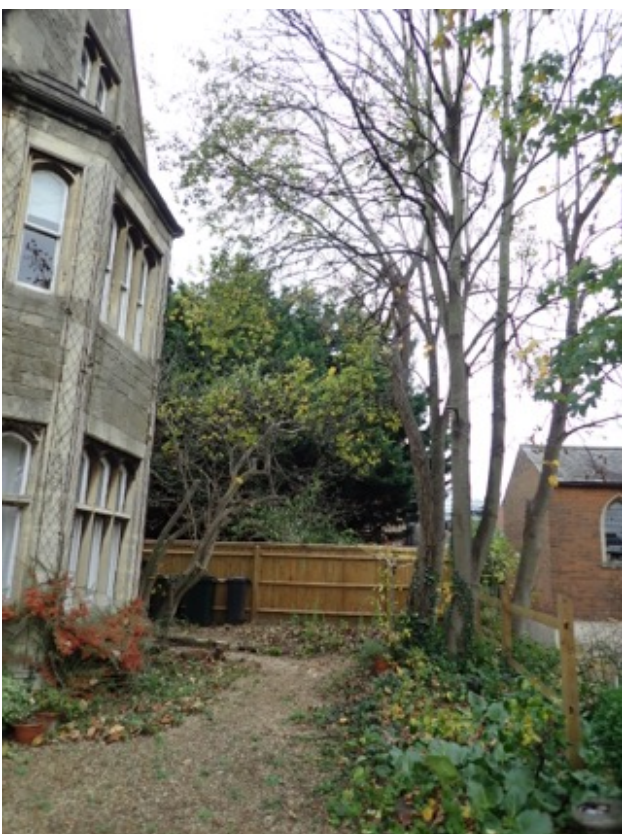
Trees outside house, at top of retaining wall. Trees are proposed for removal.
