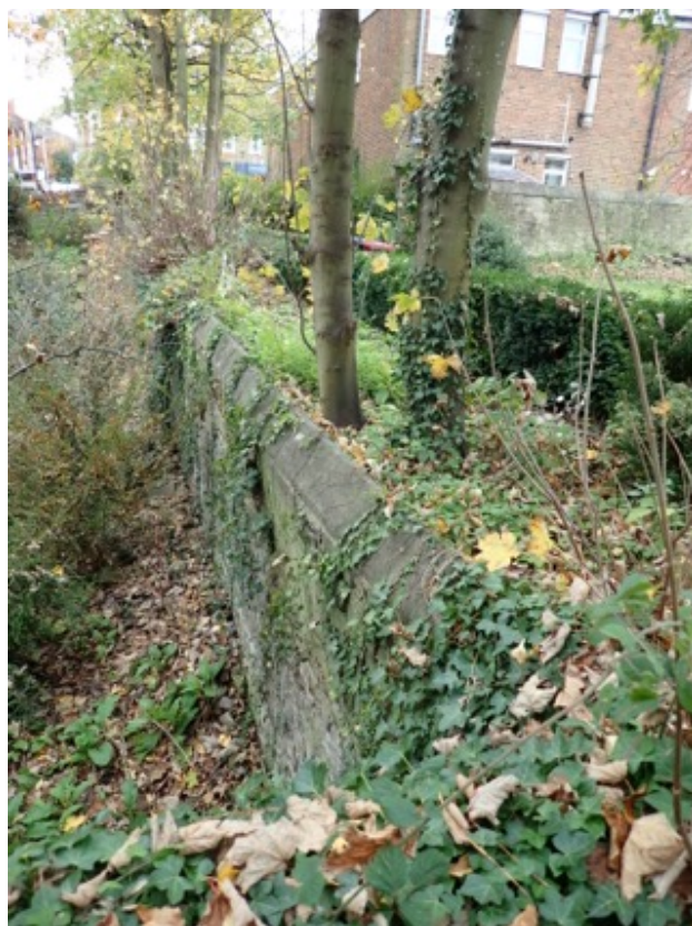
View of retaining wall between site and Holy Trinity Church.
