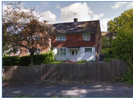
Fig 4. Front of 143 Blagdon Road. Image captured in May 2014. Image retrieved from Google Maps on 25/11/2022
