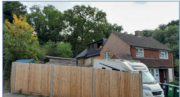
Fig 2. Rear of 143 Blagdon Road. Photo taken by case officer on 03/10/2022.
