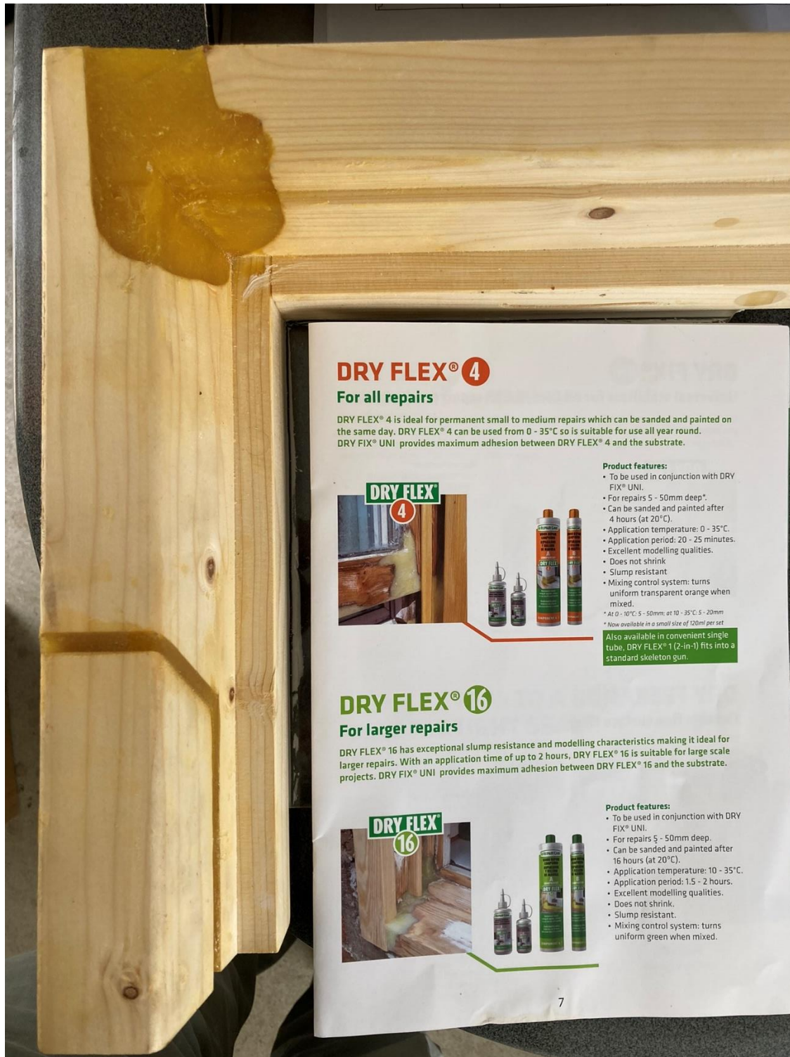
Window frame resin repairs training piece. Maximises retention of original fabric. Thick joints reduces risk of failure at joint.
