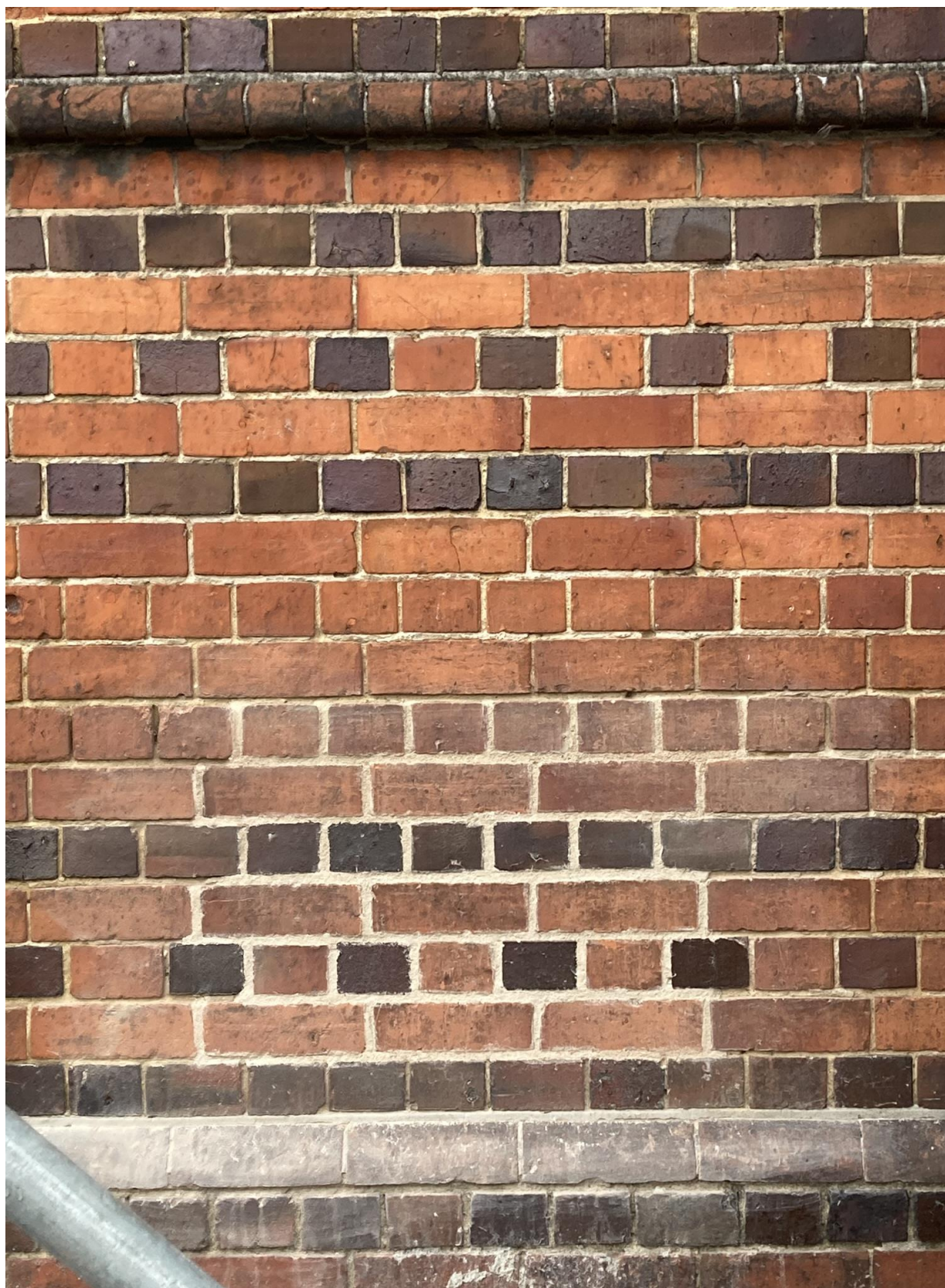
Sample of re-pointing using Morestead sand with NHL 3.5
