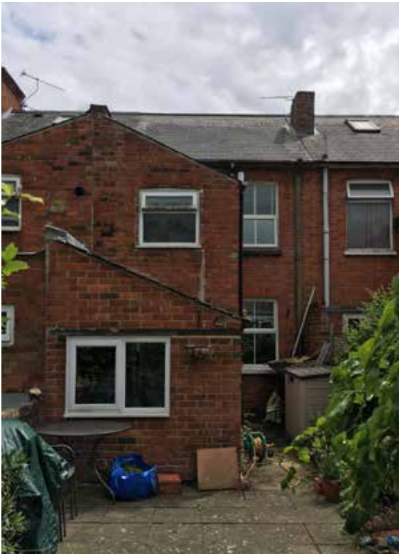
Figure 4: Photograph of existing rear elevation
