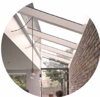
Sloped skylights to side extension
