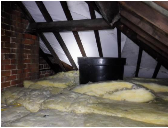
13. Internal view of the roof space.
