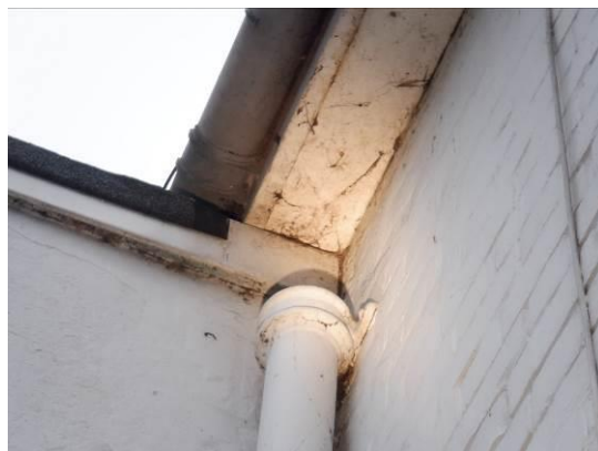
8. Timber soffits flush against the brickwork.
