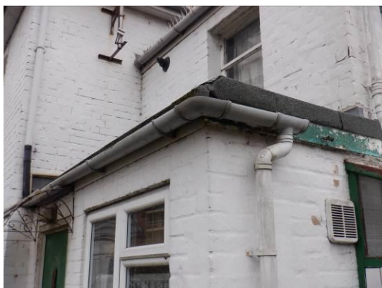
11. Section of flat roof lined with bitumen roof at the western end of the property.
