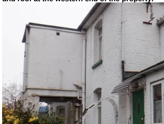
12. Flat roof extension covered with bitumen roofing felt.
