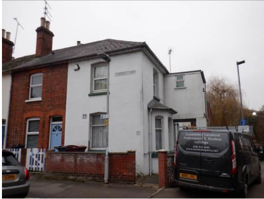
1. Northern and eastern sides of the property viewed from north-east.
