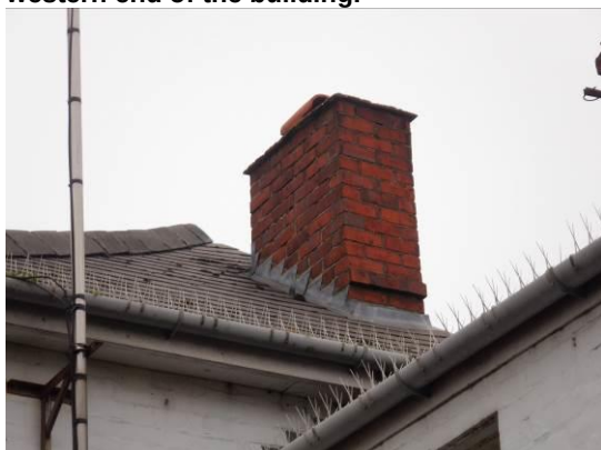
9. Lead flashing tight around the central chimney.
