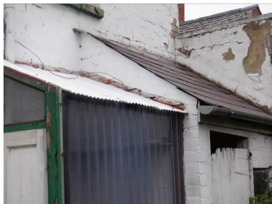
10. Toilet block with a sloped slate roof, and a bin storage area with corrugated plastic wall and roof at the western end of the property.
