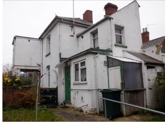
2. Northern and western sides of the property viewed from the north-west.
