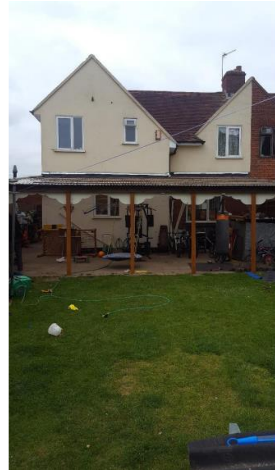
An image of the rear elevation of the property
