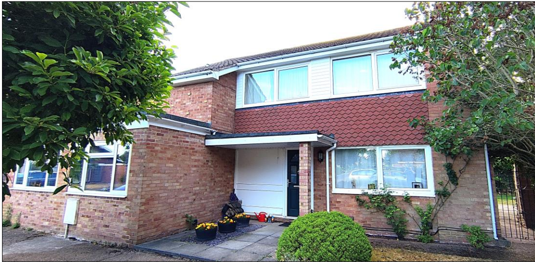
Figure 2 – Front (western) elevation of 16 Tower Close with extension to front and side
