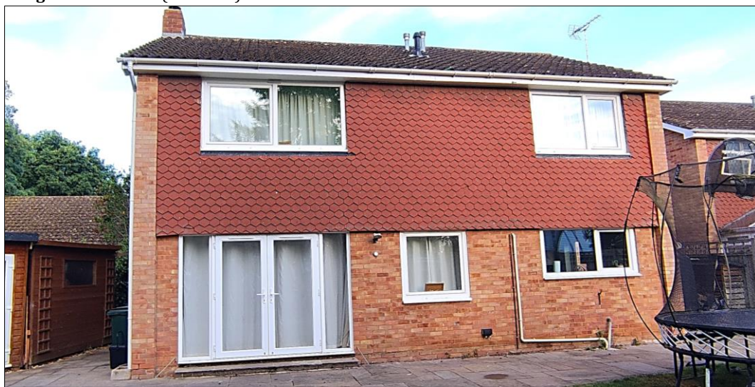
Figure 3 – Rear (eastern) elevation of 16 Tower Close hanging tiles on upper section
