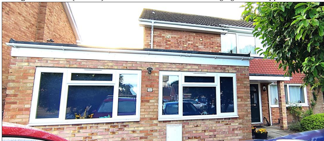
Figure 4 – Front (western) elevation of 16 Tower Close showing current wraparound single storey extension
