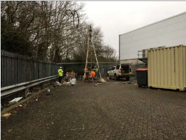
17: Cable percussive rig set up
