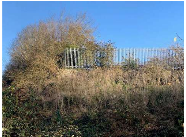
24: Overview of slope
