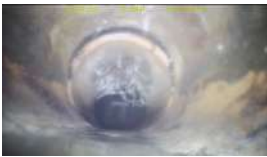
Displaced joint
