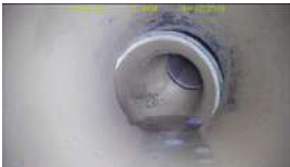
Displaced joint
