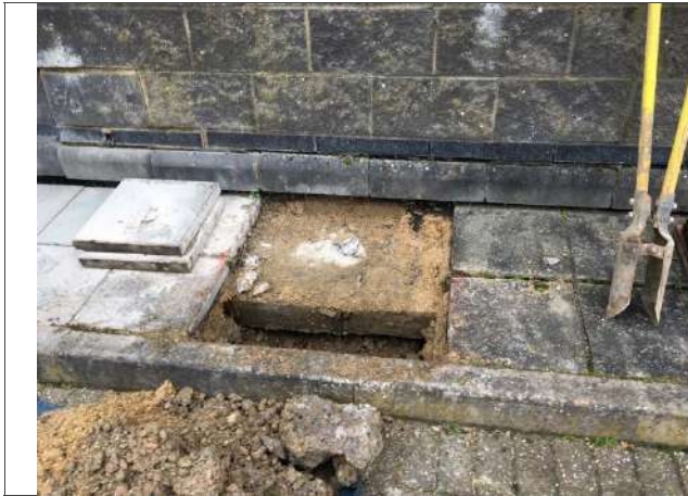
13: Exposed concrete beam
