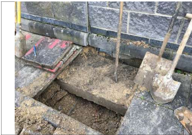
15: Continuation of concrete beam
