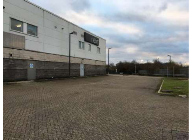
02: Rear yard overview
