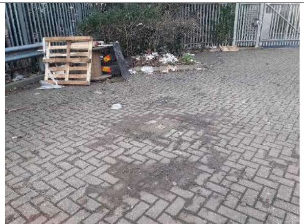
20: Example of reinstated position
