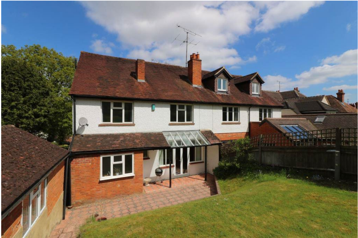
Fig. 5 Rear Elevation 21 Oak Tree Road and 19 Oak Tree Road property seen on the right
