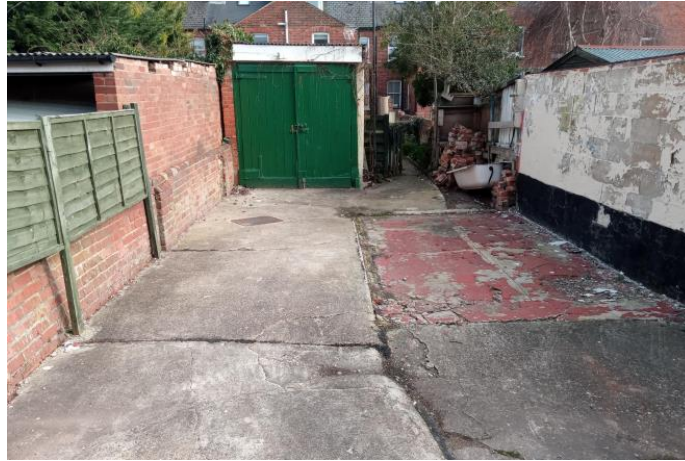
View of the existing single garage structure at No. 14 Wantage Rd & hardstanding
