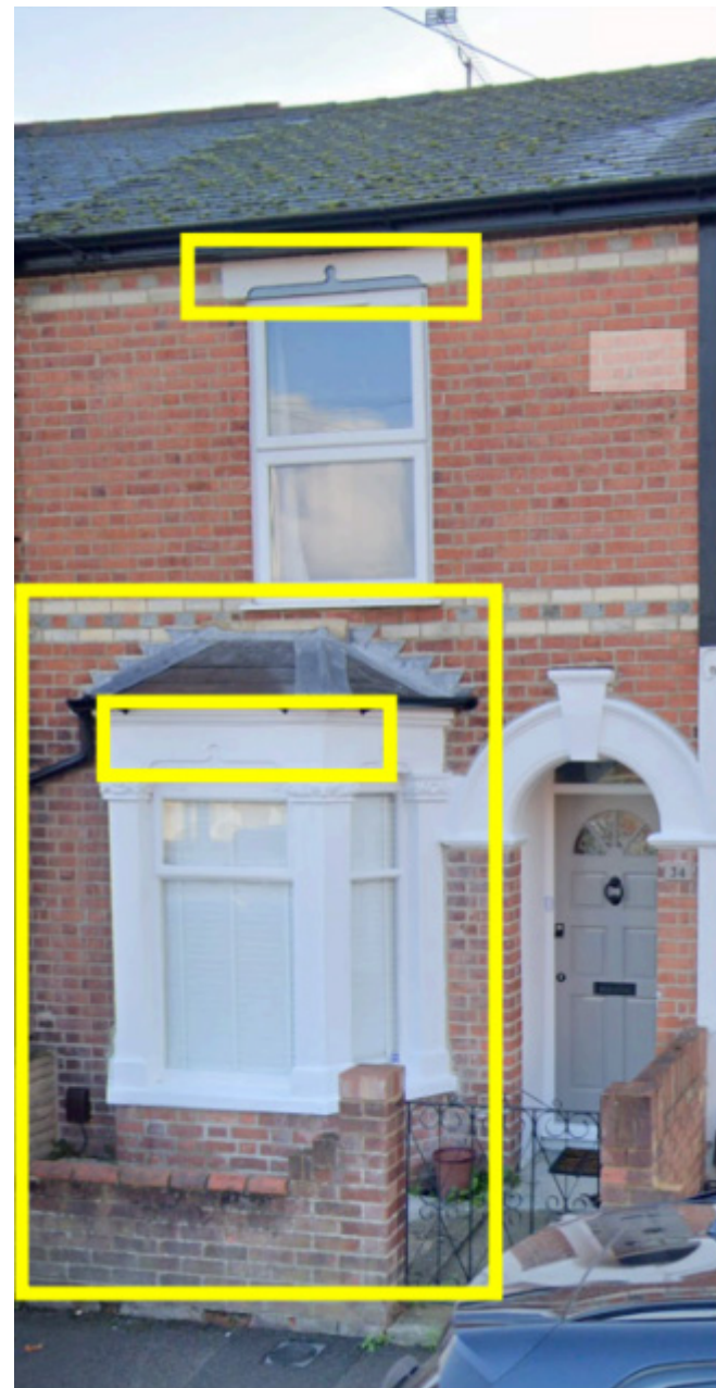
Photo of 34 Kings Road front facade, with common decorative and bay window styles highlighted in yellow.
