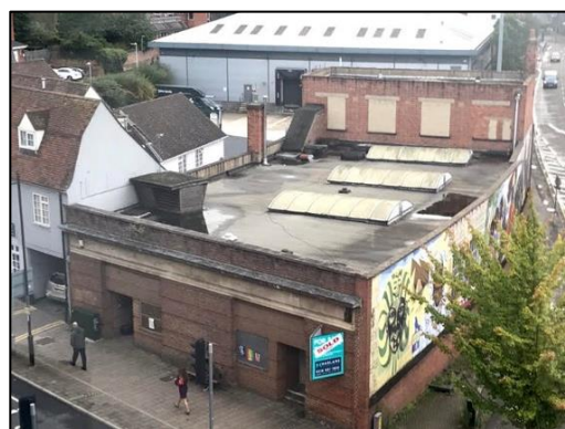
Figure 2: Exterior view showing flat roof of Central Club behind parapet
