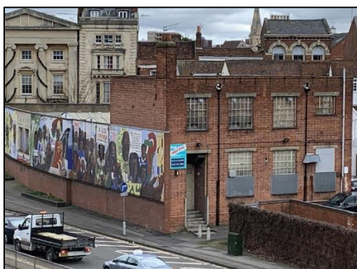
Figure 1: Exterior view of Central Club
