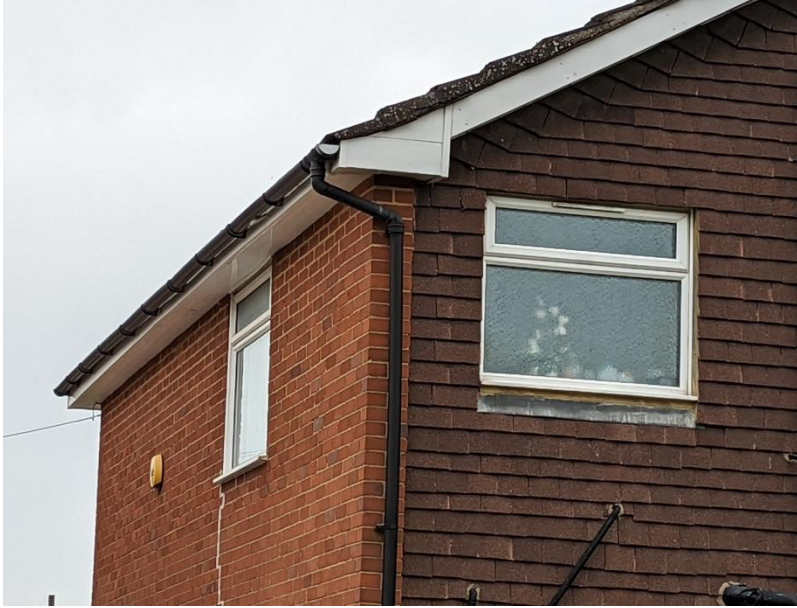
Photograph 3 – South East Elevation
