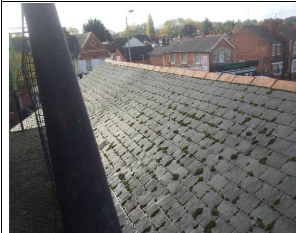
Photograph 5. The tight-fitting slate roof tiles cladding all parts of the pitched roof at the site.
