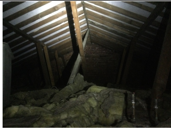
Photograph 4. The timber framed roof void within the central, two story section of the building.
