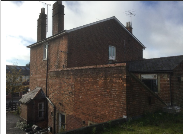
Photograph 3. The eastern facing section of the building.
