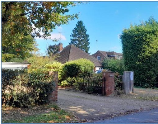
1. Front of 21 Derby Road. Photo taken on 10/10/2022.
