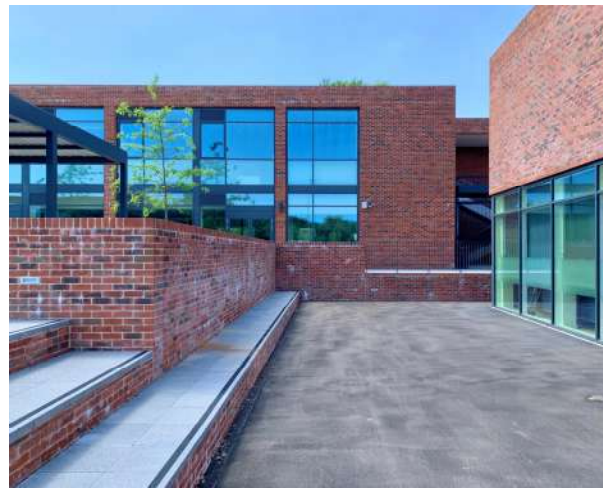
EL-5 Brick Light – To 1 st , 2 nd , 3 rd floor external terrace perimeter wall parapets
